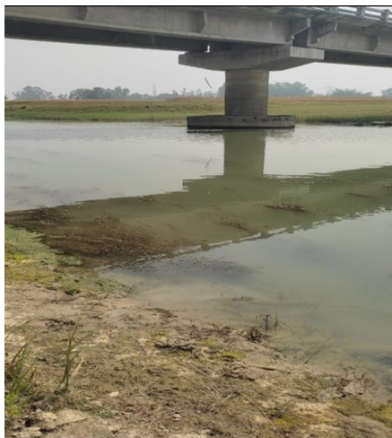
Site-4 (200 Meter Down Strem)
